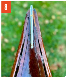
The rot was excavated and the missing material was filled with custom-fit mahogany. FIG. 8
