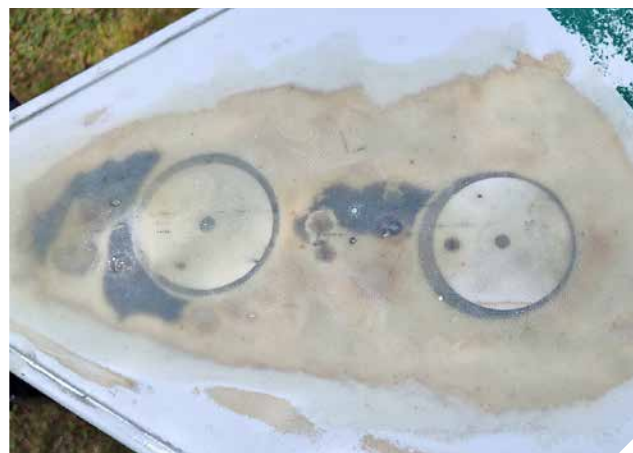
Two holes were cut in the deck to bond in a backing plate for the lifting handle.
