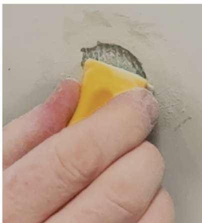
Sanding a fiberglass patch to prepare for bonding.
