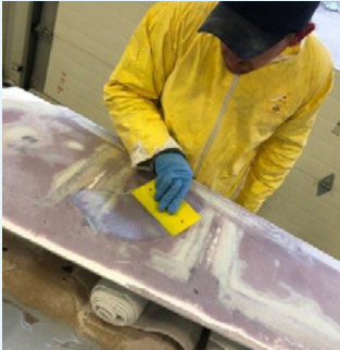
Epoxy is poured on the repair and fair'd to a uniform surface.
