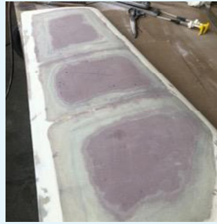
Surface is sanded in preparation for epoxy.
