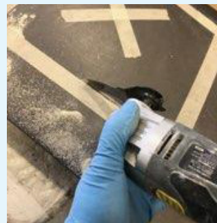
Vibrating multi tool cutting fiberglass laminate.
