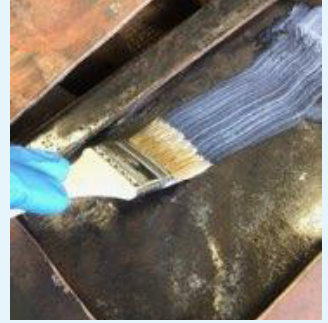
Brushing on rust convertor called Correseal®.
