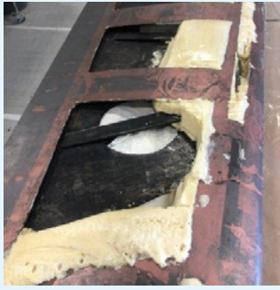
Expanded foam is cut with multi tool to remove sealed surface.
