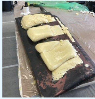
Expanding foam is poured over the surface and expands above the surface of the rudder.
