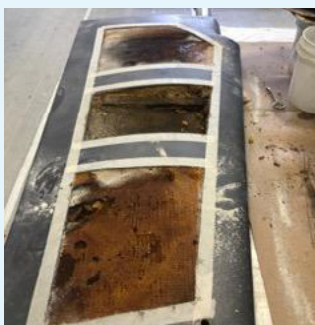
All three sections of laminate removed.
