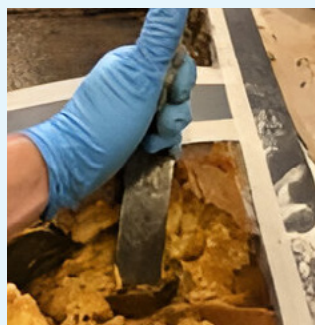
Removing foam with wood chisel.
