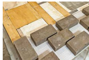
Cement blocks used compress the boards into the thickened epoxy.
