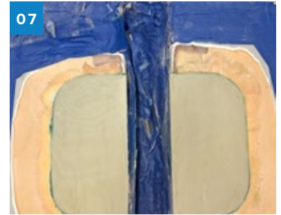
07 5/8" G-10 panels were bonded to the deck with Six10 Thickened Epoxy Adhesive.
