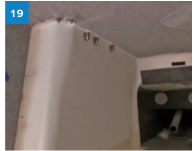
The repair finished with paint.
