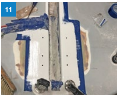
11 The repair area was taped off before applying white paint.
