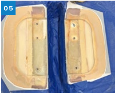
05 The fiberglass laminate was beveled around the perimeter of the cutout area. The foam was removed under the G-10 panel although some foam remained when this image was taken.
