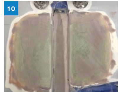
10 The 105/206/407 fairing compound cured, sanded smooth and ready for paint.
