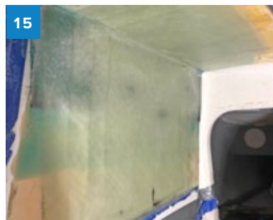
15 Four layers of 1708 were applied over the panels with 105/206.
