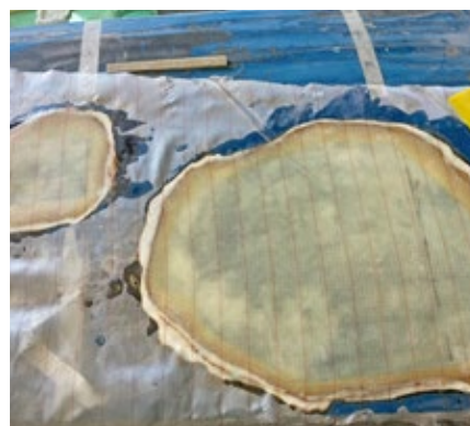
Fiberglass in place with release fabric.
