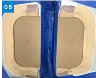
06 Thin cardboard was used to make a template for cutting the G-10 panels.
