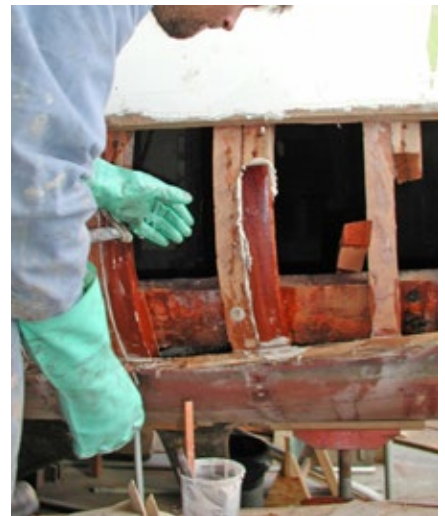
With every rib in the boat inspected, we used mahogany laminate strips and epoxy to repair the ribs. We used laminations to repair the bilge stringers where they were inaccessible under the bulkheads. Longer, accessible stringer sections were repaired with new boards and long scarf joints with epoxy. Where stringers had oversized holes caused by bolt corrosion, we double plugged the holes with epoxy and installed a new silicon bronze bolt.
