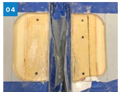
04 To make room for the G-10 panel, I removed the high-density foam with a router.
