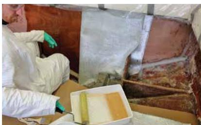
*Applying fiberglass to the plywood transom.*
