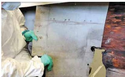
*Removing the inner skin from the rotten plywood.*
