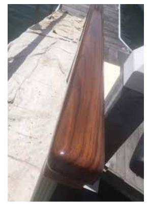
Three coats 105 Resin/207 Special Clear Hardener and two coats of two-part polyurethane
