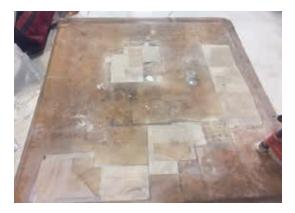
Multiple areas had damaged core and needed replacement.
