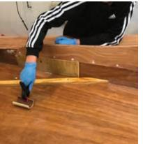
After brushing the epoxy on, Joshua tipped the coat with a section of a 300 Roller Cover with a clamp for a handle.
