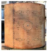
The drum has been stripped in preparation for the repair.
