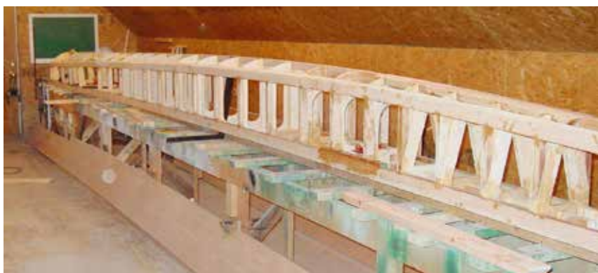
Michigander's fuselage being built in Yaeso's second story workshop in Green Bay
