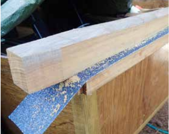
36-grit sandpaper helps create a lot of tooth for the epoxy to grab onto.
