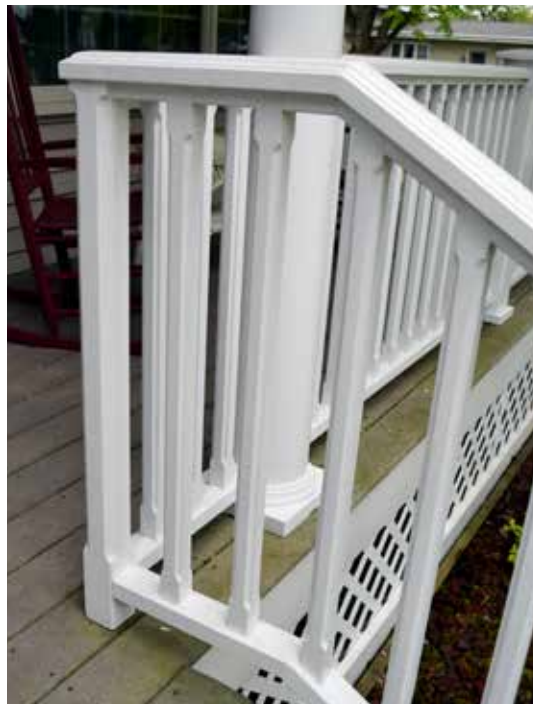
The freshly repainted railing with its decorative fluted spindles.
