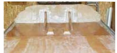
Deck, transom knees, and fuel tank mounts after glassing with bi-axial fiberglass and WEST SYSTEM Epoxy
