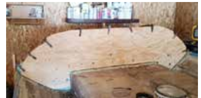
Two-ply of 3/4" marine grade fir bonded to transom
