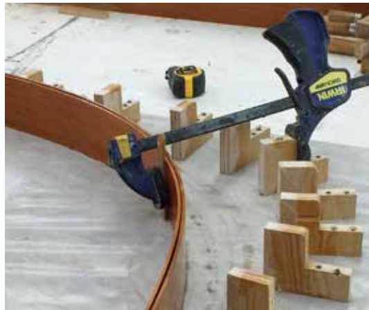
The jig fixture we built for the two front trim pieces with one new piece almost pulled into shape.
