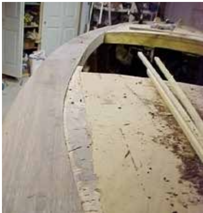
Walnut covering board in place
