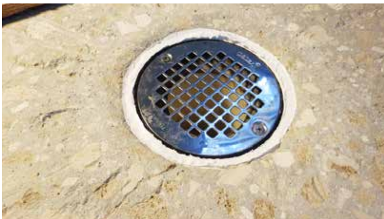
The finished drain installed.
