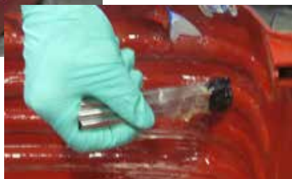
Right: three brushes are taped together to expedite the wetting out process.
