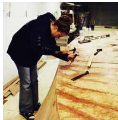
Mark's daughter removing staples from the hull after its second layer of planking.
