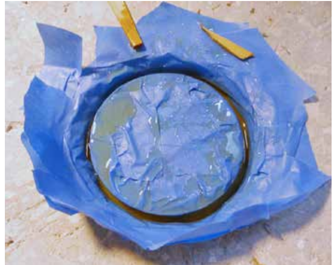
The G/flex 650 collar poured and curing.
