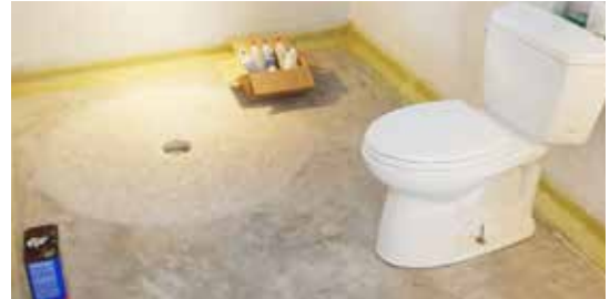
The beveled slope to the shower drain.
