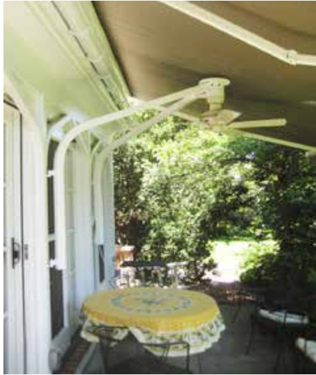
The fan with support crane installed and awning extended.
