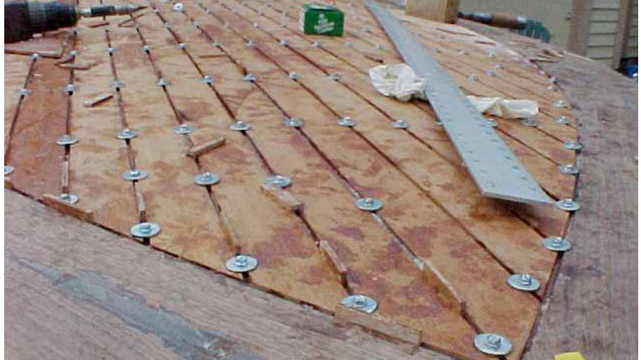
Mahogany planks were epoxied onto the deck. Once the screws were installed, the temporary plywood spacers were removed before the epoxy cured.
