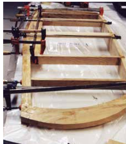
The transom assembly coated with epoxy to prevent water intrusion.
