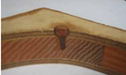
Note cutaway of hole and plug how all the end grain that the screw exposes is protected with epoxy.
