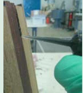
After sanding, fill any voids with unthickened pigmented epoxy
