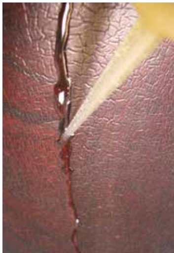
Left: Warming the repair area with a heat lamp. Center: Epoxy applied to the crack through a syringe. Right: Removing excess epoxy smears with cheese cloth.
