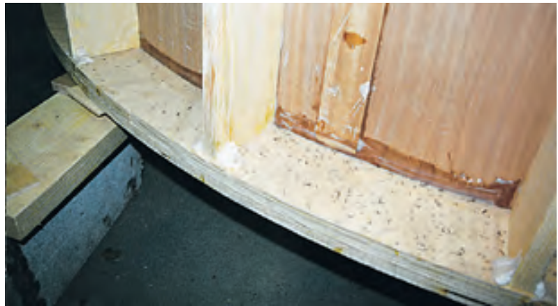
Above—Detail of the back of the wall showing 1"×4" studs, two" plywood plates and a plywood butt block. Keep the butt block 1½" shorter than the plywood panel on each end, so it will clear the top and bottom plate.
