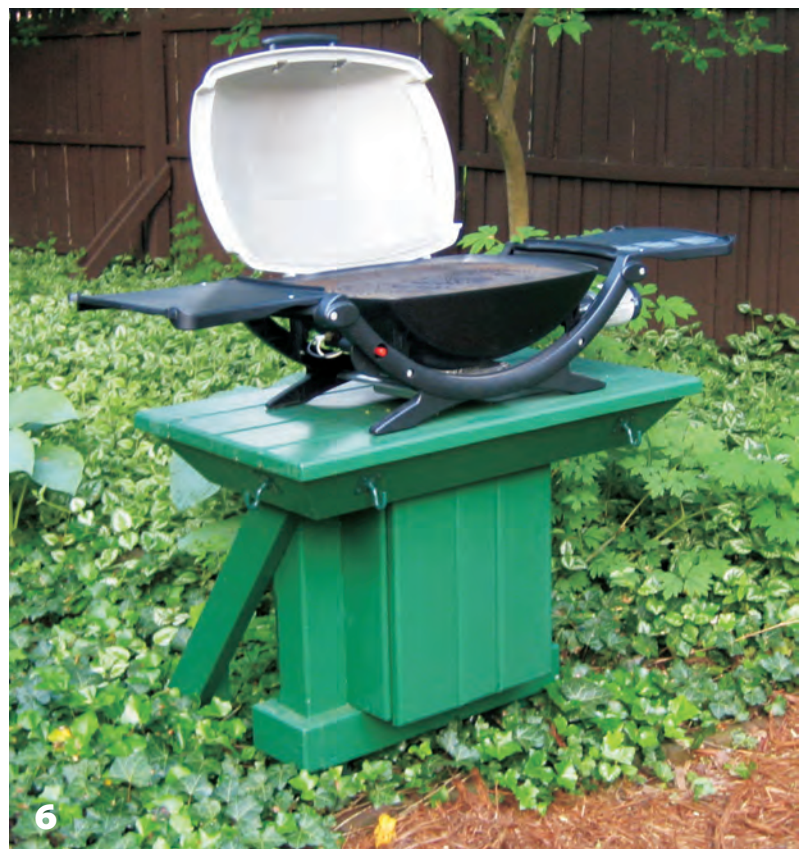
Figure 6—The table was secured in the earth with four 30"x4"x4" METPOST™ fence supports. The back-reaching legs, held down by the clamping collars of the fence supports, produced stability for the forward extended table top.
