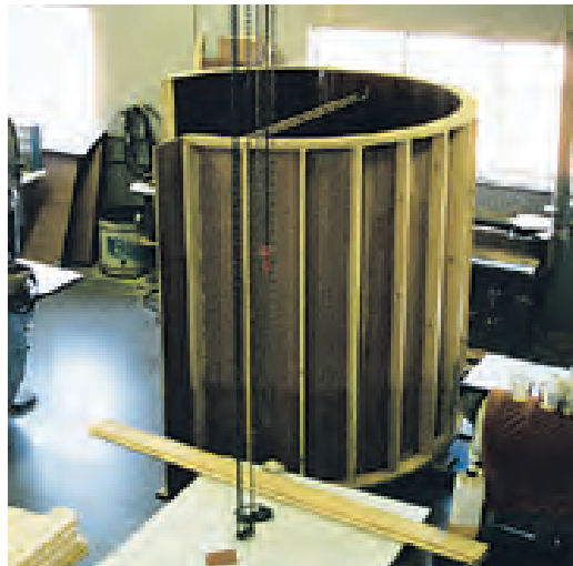
Above—Detail of the back of the wall showing 1"×4" studs, two" plywood plates and a plywood butt block. Keep the butt block 1½" shorter than the plywood panel on each end, so it will clear the top and bottom plate.
