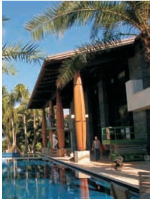
The finished 24' front columns built by Pleasant Bay Boat and Spar Company.
