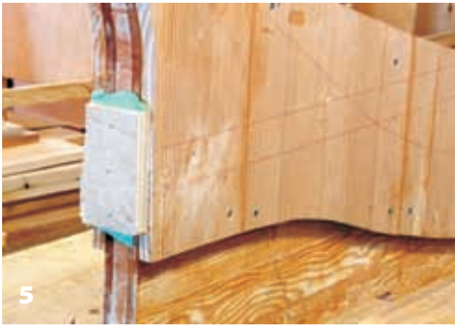
5. We reassembled the core by gluing the first layer on one side using the screw holes as a guide.
