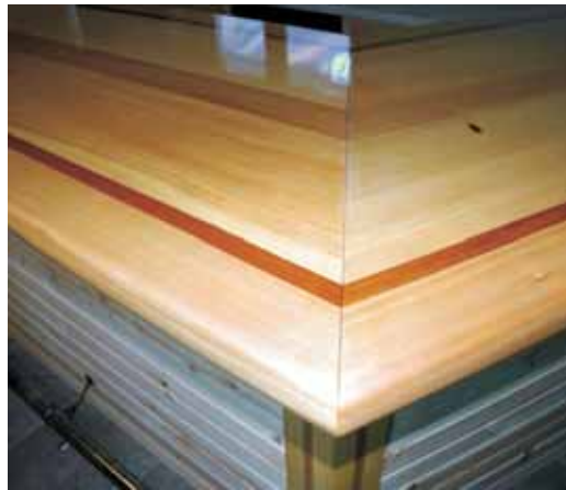
The corner detail showing the Sitka spruce field with mahogany accent strips. The top has four coats of 105/207 wet sanded between the third and fourth coat.
