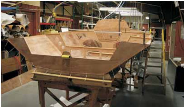
Left—With all of the bulkheads in place the ties were cinched tight before fillets and fiberglass tape were applied to reinforce the joints.
