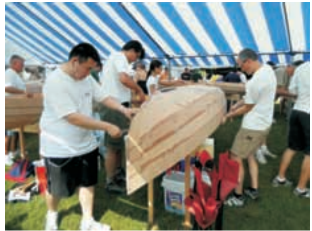
On day two the bottoms of the interiors were fiberglassed. The now rigid hulls were rolled over and the copper stitching was removed.
