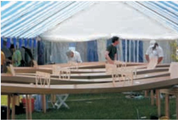
Temporary and permanent bulkheads are wired in place. By the end of day one, all of the strakes were stitched in place and the laps were glued with Six10 Adhesive.
