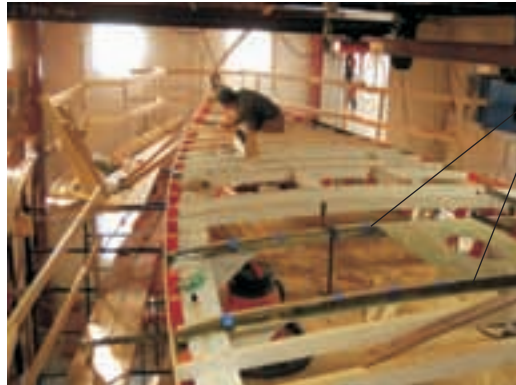
Deck frames being installed with the Monel weldment visible.
