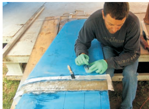
Repairing cracks on the side of the rudder with WEST SYSTEM Epoxy and fiberglass cloth.
