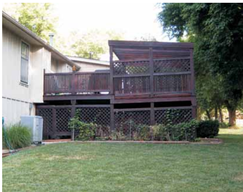
Blackmon's two-story deck is supported by 6×6 redwood posts resting on concrete footings.
