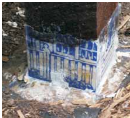
The forms were removed from the cured epoxy revealing the ink that transferred from the inside of the form to the epoxy.
