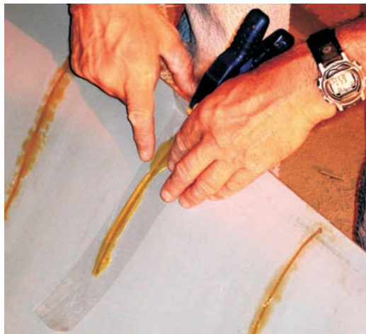
Stan running tape over freshly glued cracks to prevent the glue from running and keep it relatively smooth when cured. Note use of simple spring clamp to keep top edge of the Royalex aligned.
