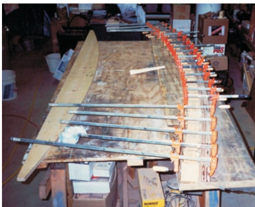
Puehl laminated the deck and cabin roof beams in a custom jig. The jig produced beams in an arc with a 21' radius.
