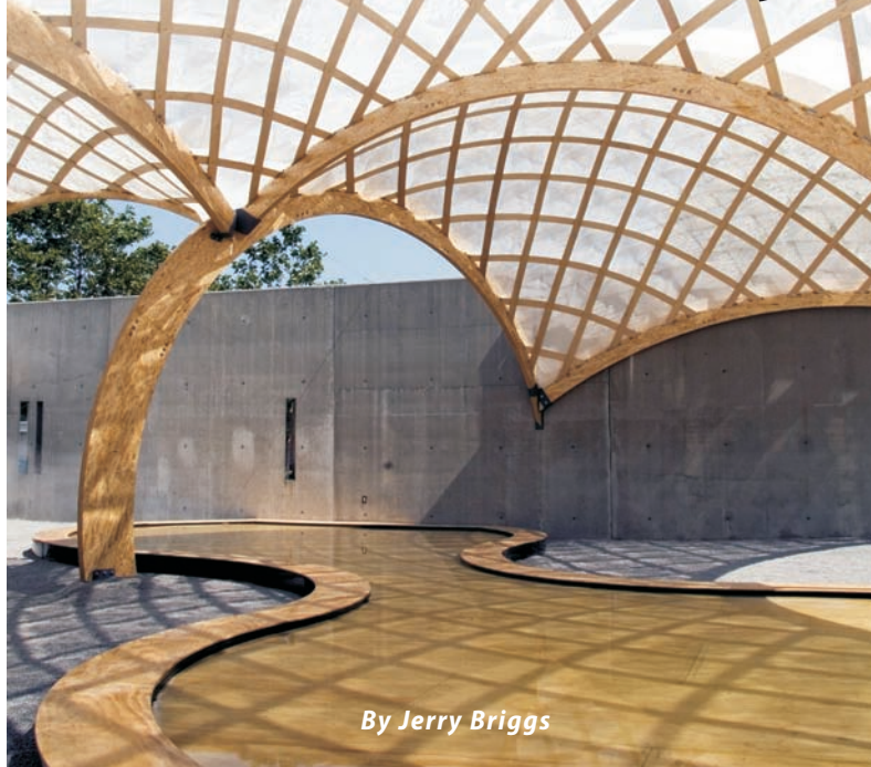
Figure 1 —A large, walled triangular outdoor gallery space was partially covered with seven shells and included two shallow tidal pools. The structures and pools were manufactured in a workshop and later deployed on site.
