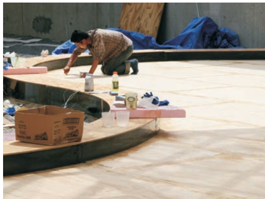
Figure 5—All of the seams on the pool bottom were sealed using 3" cloth tape and three coats of epoxy.
