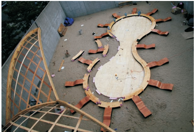
Figure 4—All sections were staged in place before they were bonded with epoxy thickened with a structural filler.
