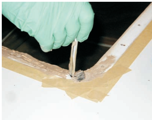
← Photo 3 —Mask off the surrounding deck with wide masking tape.
